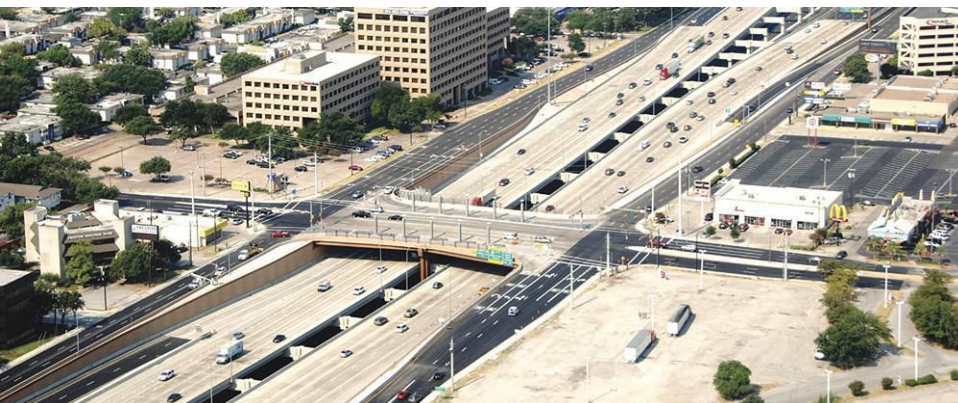
The cantilevered design of the TEXpress lanes in the center of the roadway saved $1 billion in construction cost.
