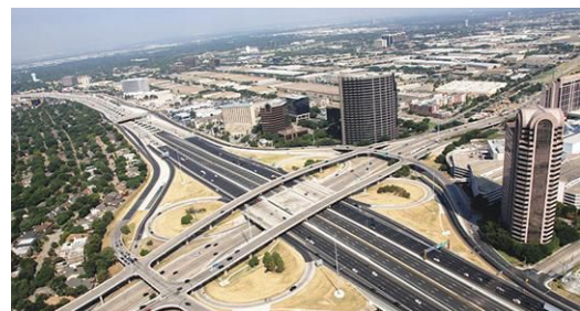
Bird's eye view of the LBJ Express after construction is complete
