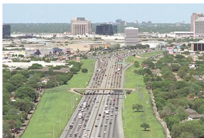
A look at the LBJ Express prior to construction
